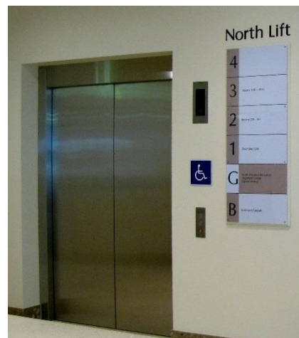
Figure 5.6: Directory sign beside lift entry
