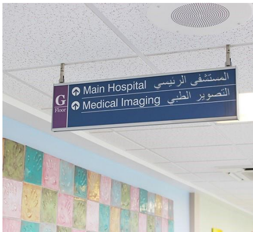
Figure 5.5: Corridor directional sign, ceiling mounted
