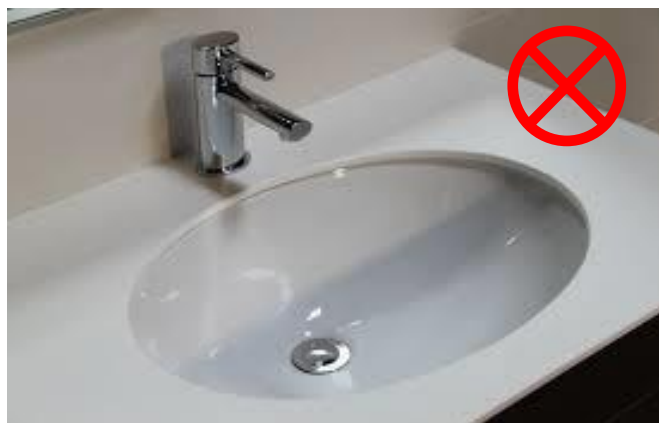
Figure 4: Under mount hand basin not recommended
