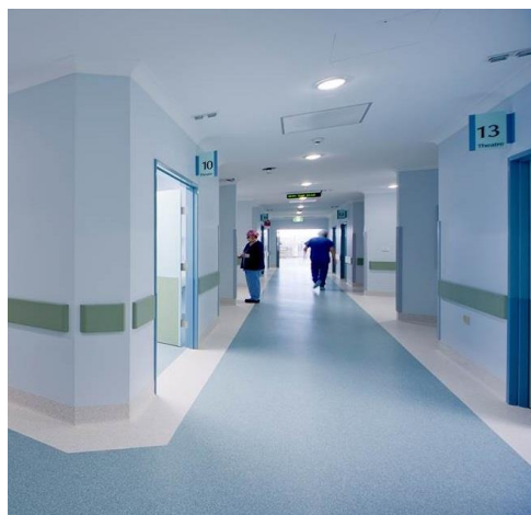
Figure 27: Seamless flooring and coved skirting in clinical areas such as Operating Unit are integral and coved
