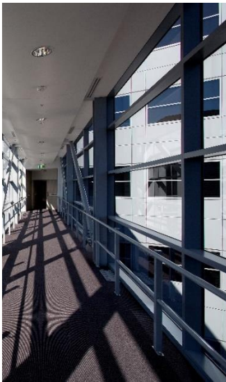
Figure 8.2: Fixed windows in corridor
