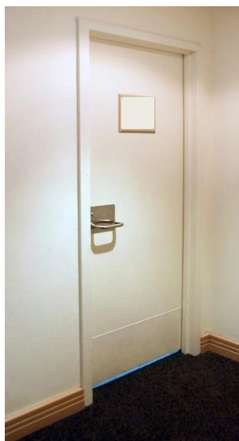
Figure 6.12: Door with undercut
