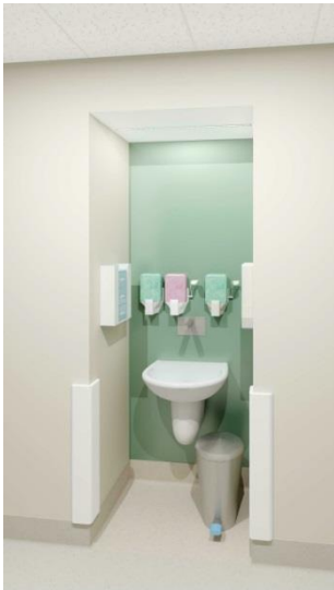
Figure 2.9: Reduced height ceiling within a corridor bay
