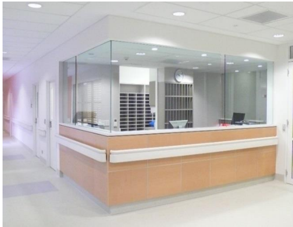
Figure 4.5: Staff Station with security glazing barrier
